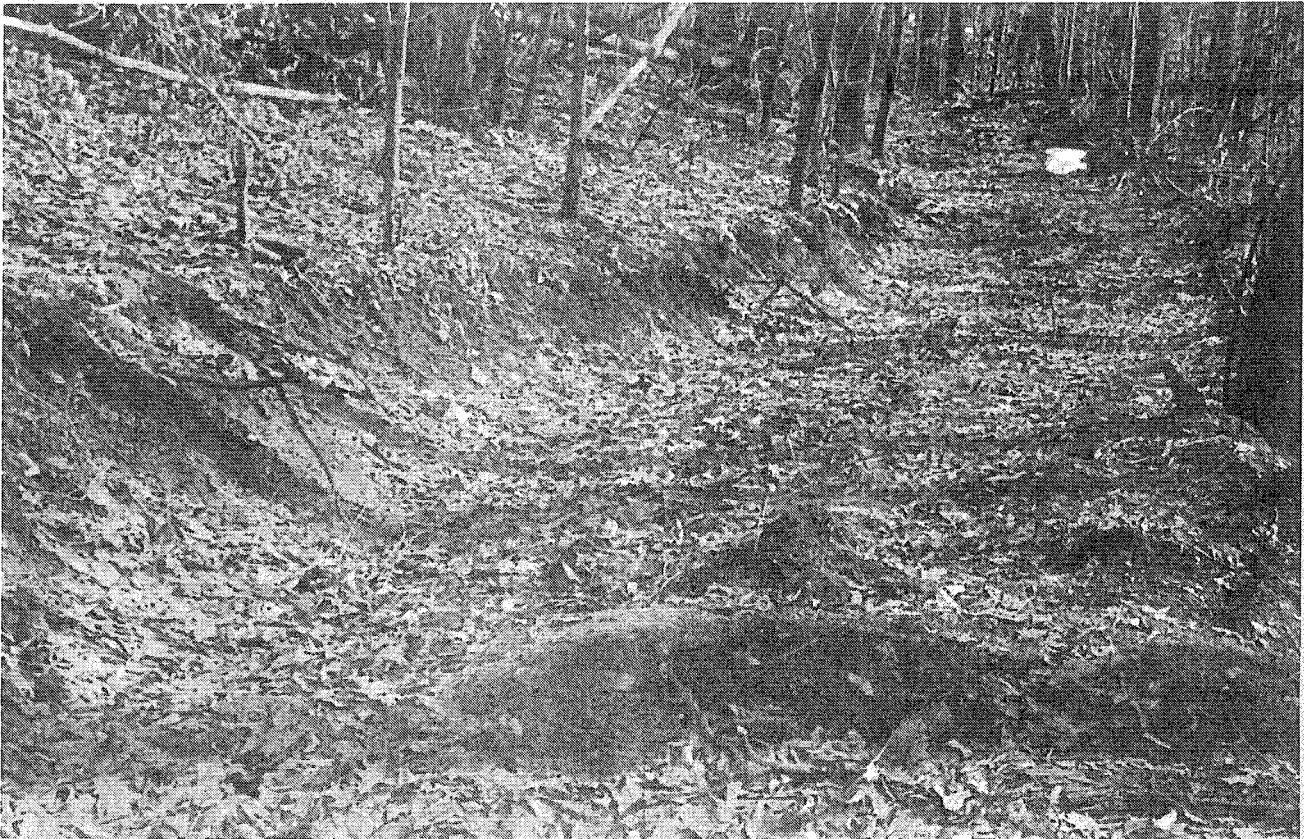
Figure 10.—Tractor skidroad in the Intensive Selection Watershed just before logging. Note the gentle grade and the dip for drainage.
