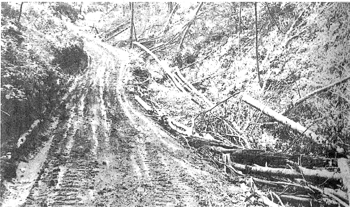
Figure 8.—Tractor skidroad in the Commercial Clearcut Watershed. The road is almost in the streambed, and logging debris obstructs the channel.
